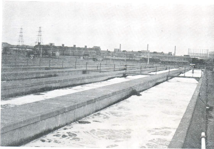
Fig. 16 — LONDRES, Northern Outfall Works — Activated sludge tank — Tanques de lodos ativados.
